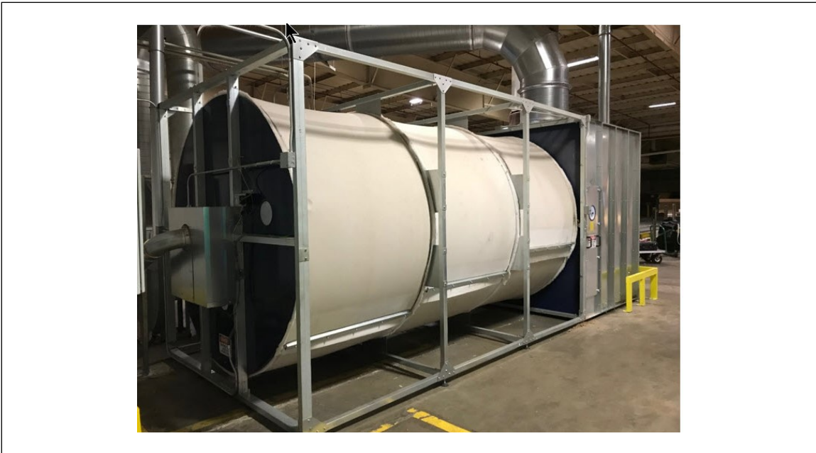
Fig. 3.4.1.2-1. Example of an enclosureless drum filter
