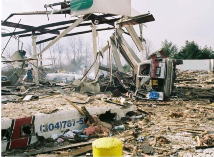
Fig. 11. Remains of a deflagration at a convenience store (Source: US CSB)
