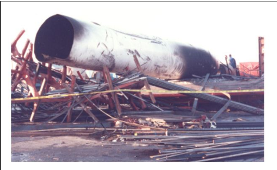
Fig. A.2. Final position of ruptured LPG tank segment
