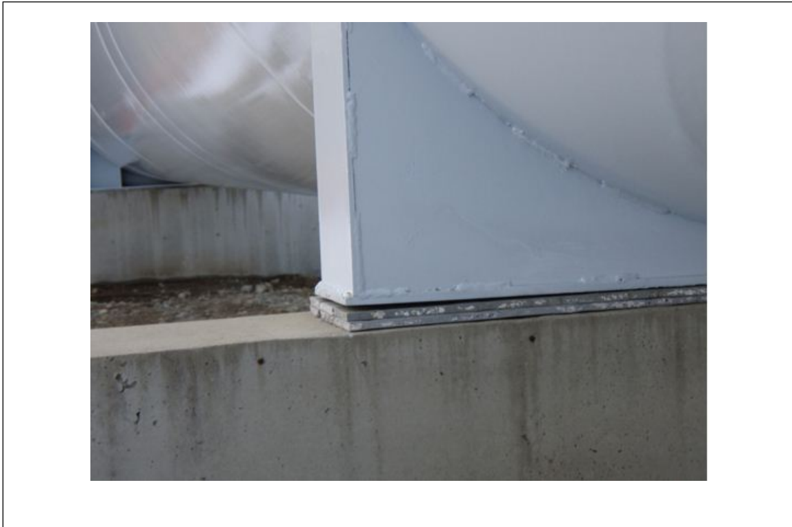
Fig. 3. Horizontal tank restraint by friction only
