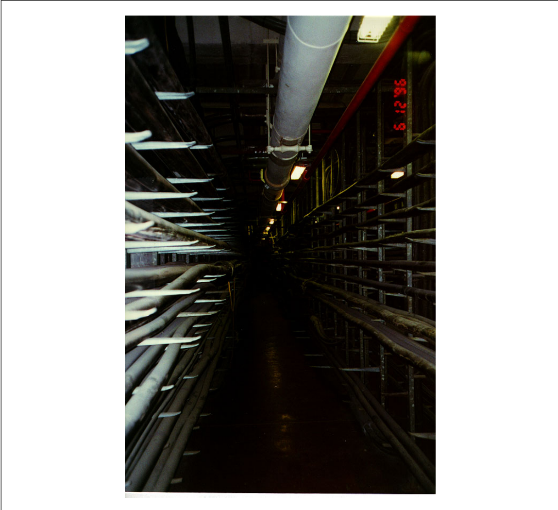
Fig. 7. Cable vault located in a large metropolitan switching center
