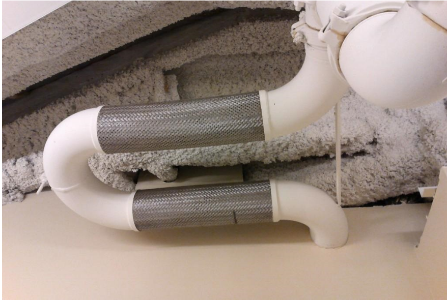
Fig. 3.1.10-B. Flexible pipe loop; possible alternative to a seismic separation assembly
