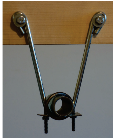
U-hanger with U-bolt retainer preventing upward movement
