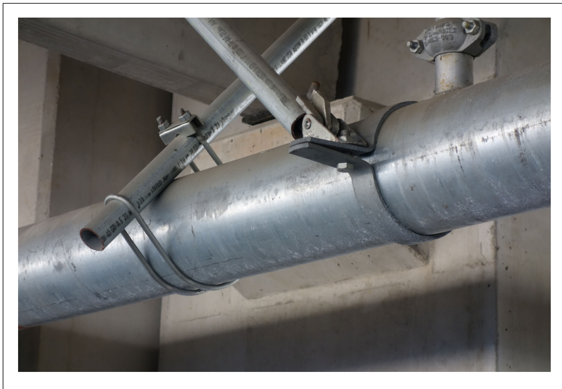
Fig. 3.1.1-B. Examples of pipe-attached components (must be FM Approved)
