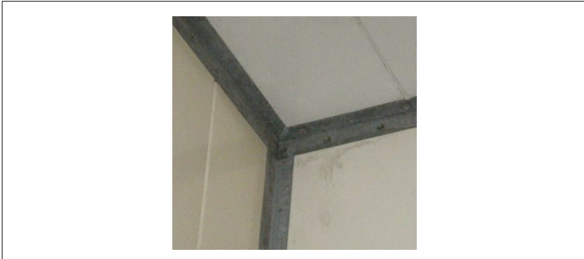
Fig. 2.2-1. Angles provided for securement
