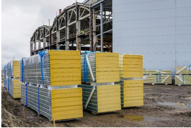
Fig. 3.2.1-1. Polyurethane foam core example (usually a yellow color)
