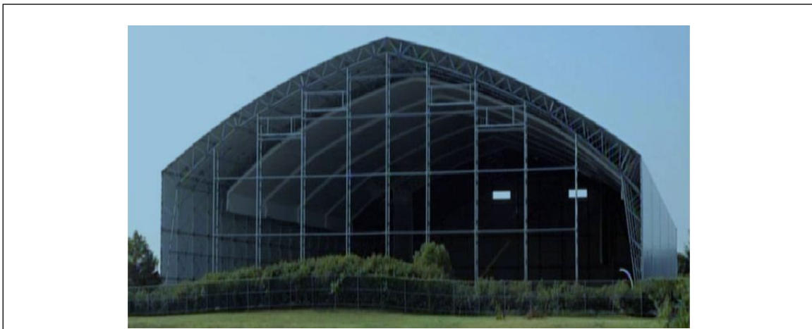
Fig. 3.1.1-3. Fabric-covered structure under construction
