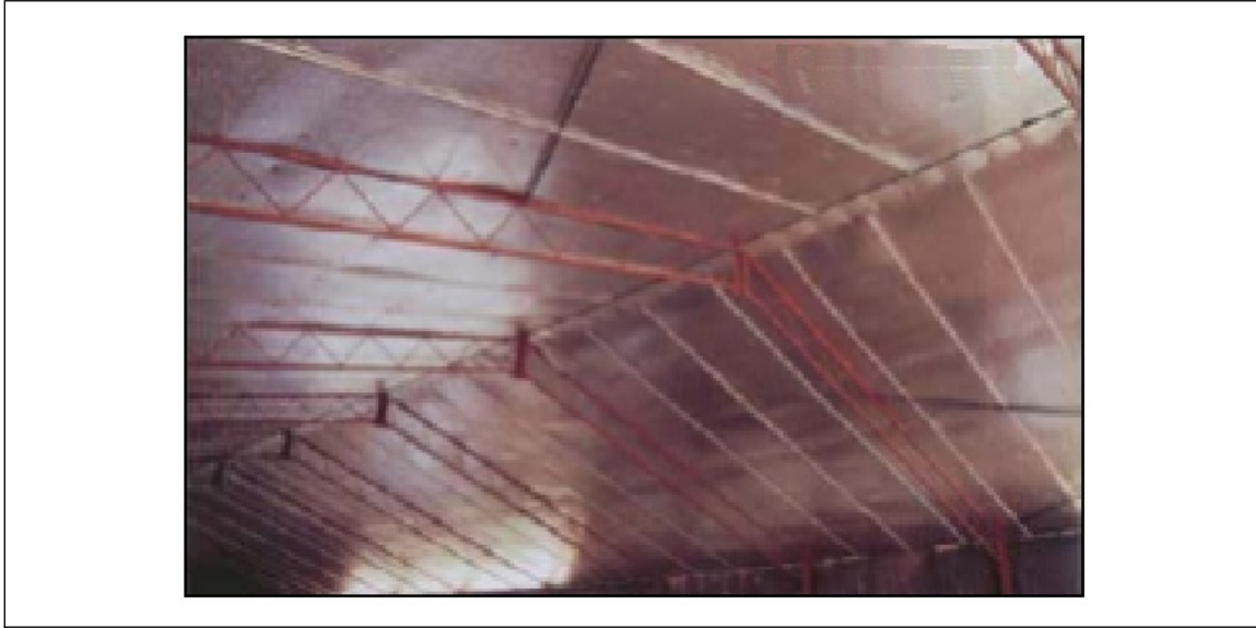
Fig. 3.1.5-1. Cross-linked polyolefin foam with factory-applied reinforced 9 \mu\text{m} aluminum foil and G60 acrylic adhesive backing
