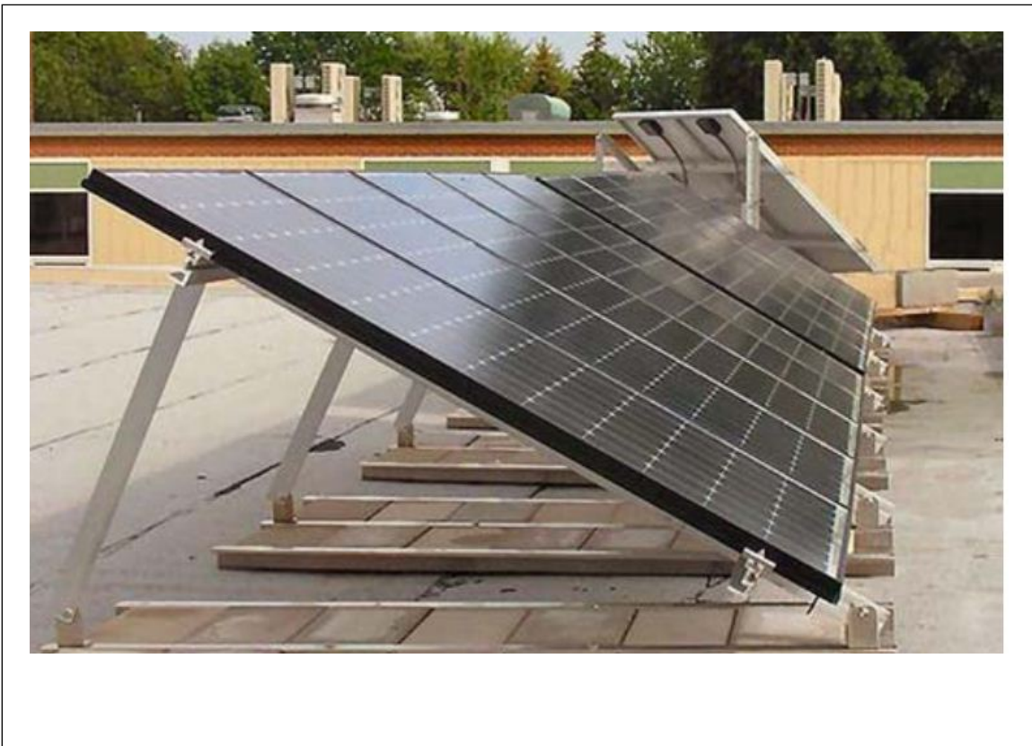
Fig. 3.2.1.1b. Solar panels with steeper slopes or lacking wind deflectors will experience greater wind effects
