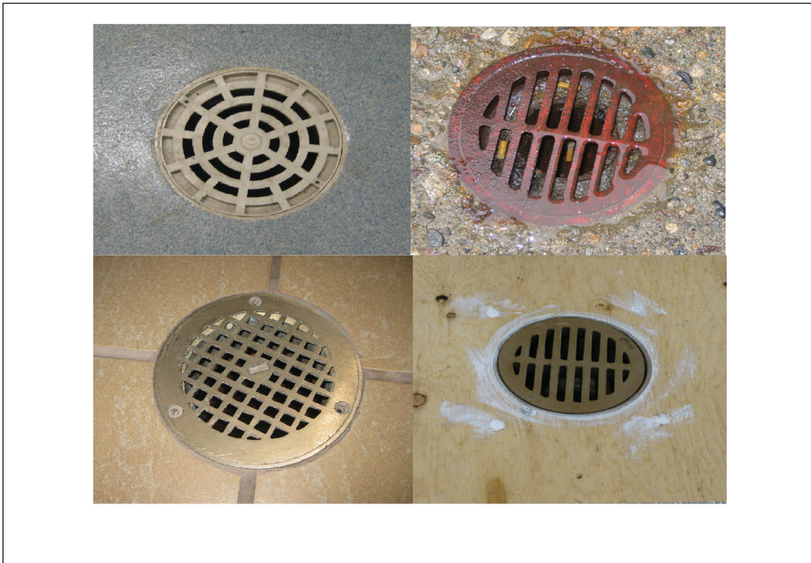
Fig. 8. An industrial-style drain grate with a free area of approximately 20-30%
