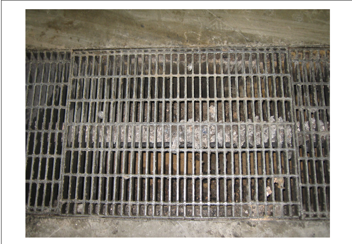
Fig. 9. An industrial-style drain grate with a free area of approximately 50%
