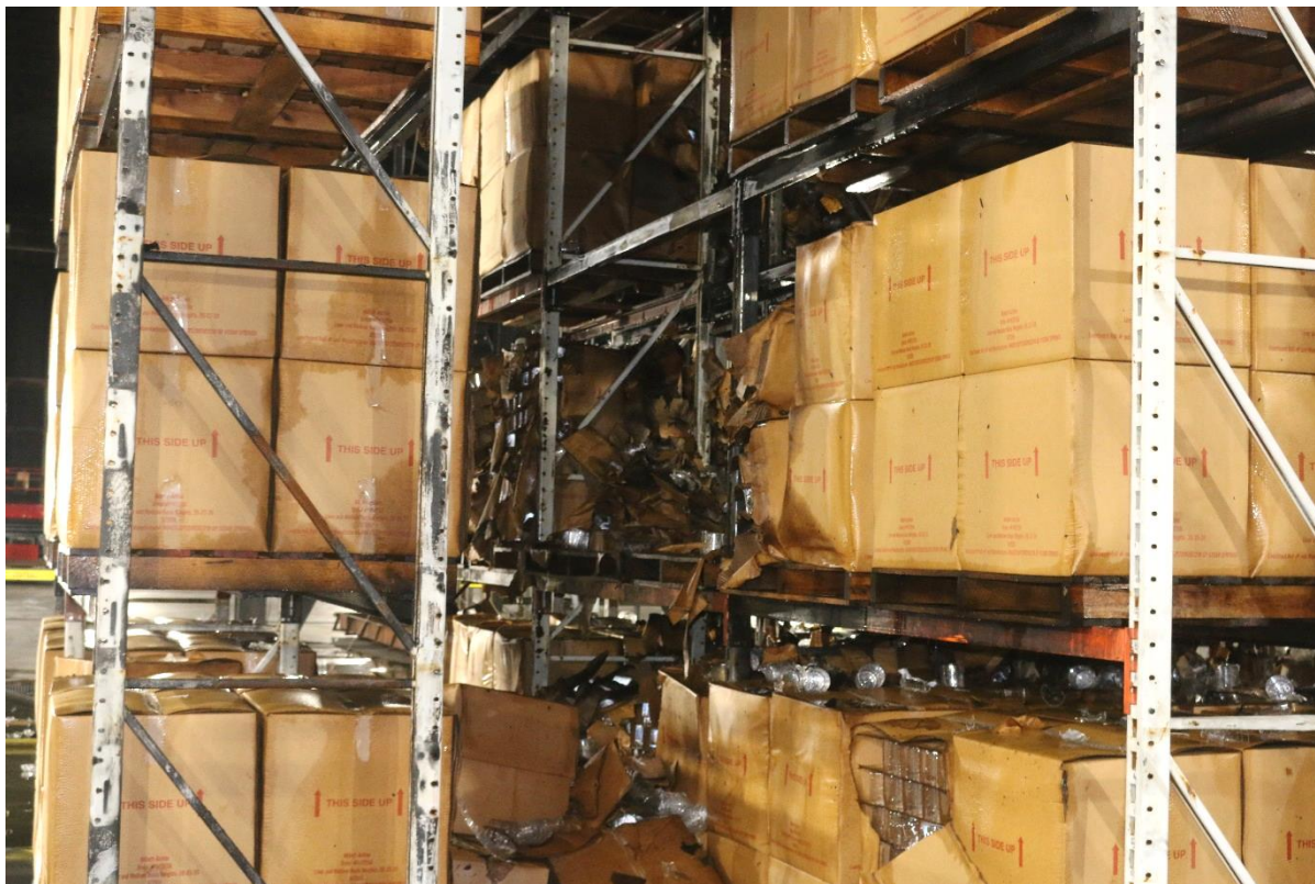
Figure E-21: Test #3 post-test close-up photograph of the east face of the main array showing fire damage.
