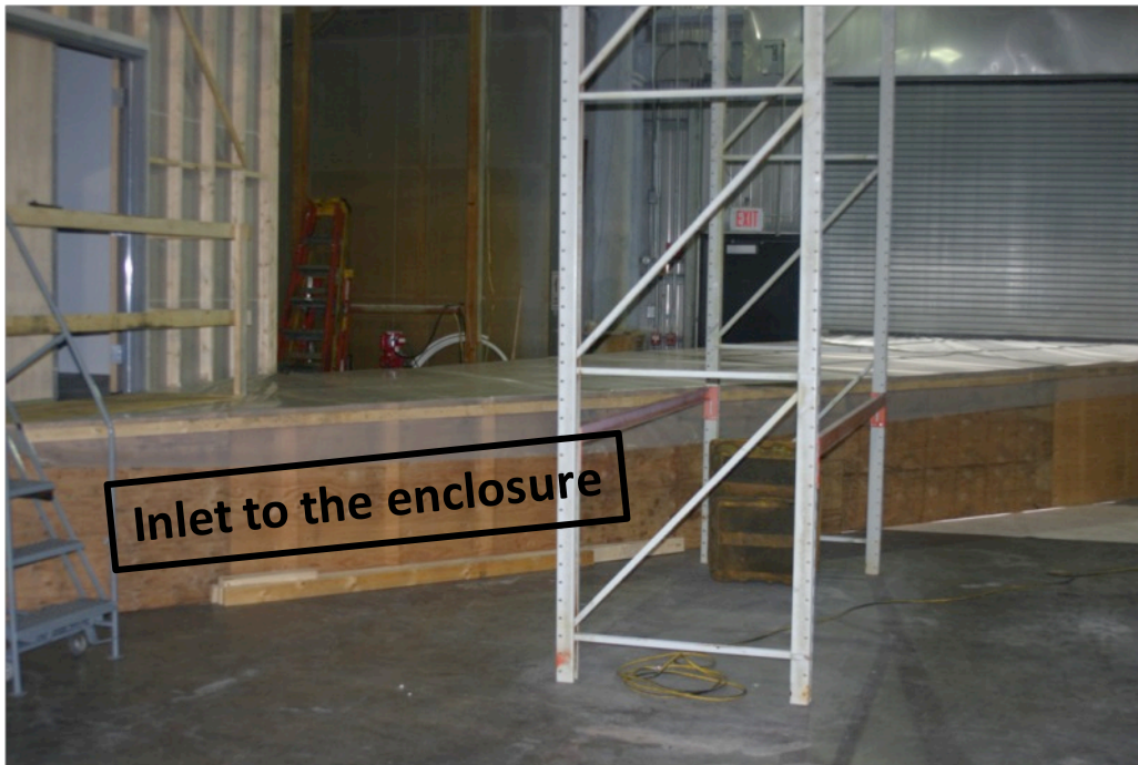
Figure 2-9: Photograph of inlet channel into the enclosure subfloor.
