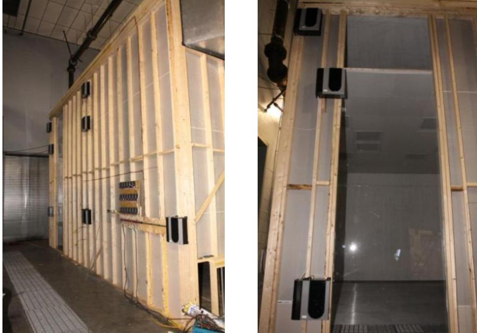
Figure 2-8: Photograph of the test enclosure south wall (left) and a close-up of full height window (right).
