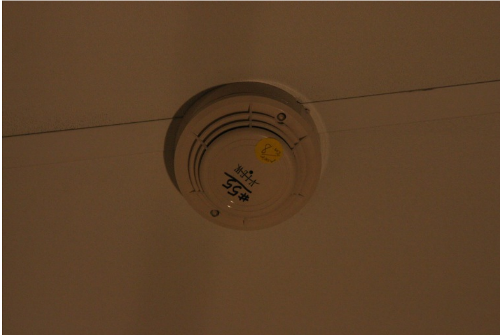
Figure 2-23: Photoelectric smoke detector (Spot-T)
