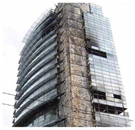
Combustible wall construction allowed fire to spread up the corner of this building.
