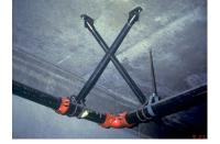
Proper bracing at change in direction
