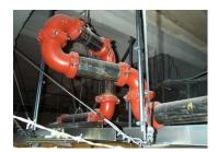
Seismic separation assembly
